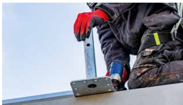
Horizontal mounting bracket
