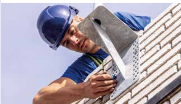
Vertical mounting bracket
